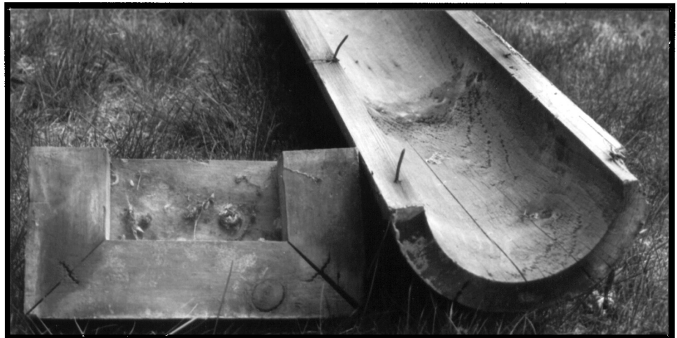
Fig. 3. One half of a hollow-bored column shaft.
