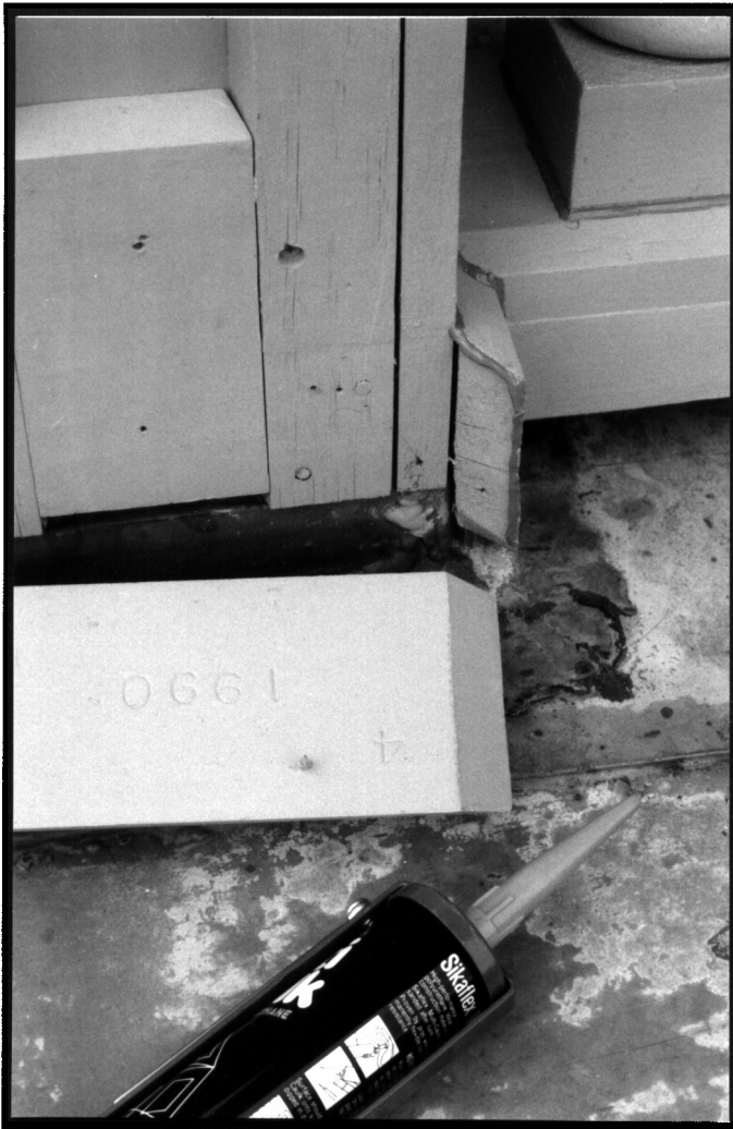
Figure 16. The miter joint of the base board is caulked into place (above). Sealant is gunned onto the miter joint just before nailing in place. A designed joint is used to seal the top edge of the base board (right).
