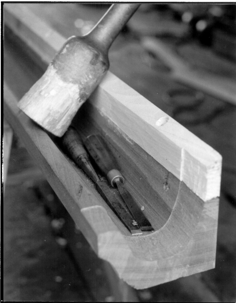
Figure 8. Depression for Flashing
