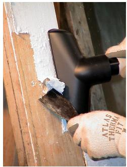
After 30 seconds to 2 minutes of steaming the paint film is soft enough to remove with a stiff, slightly dull putty knife. This paint film stays soft for 10 to 15 seconds, which is plenty of time to remove a 3" x 9" area of paint. During removal the steam head is shifted over to the next section.
