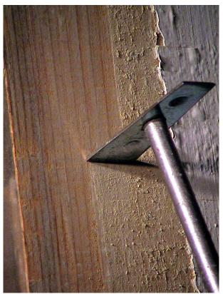
This paint film is about as thick as a dime (.035"). You can see there is some slight paint film residue left on the surface, which is easily scraped off with a sharp pull-type paint scraper while it is still soft. The result is a smooth clean surface ready to paint. Every paint removal project has different paint and wood conditions, so the procedure and results vary.
